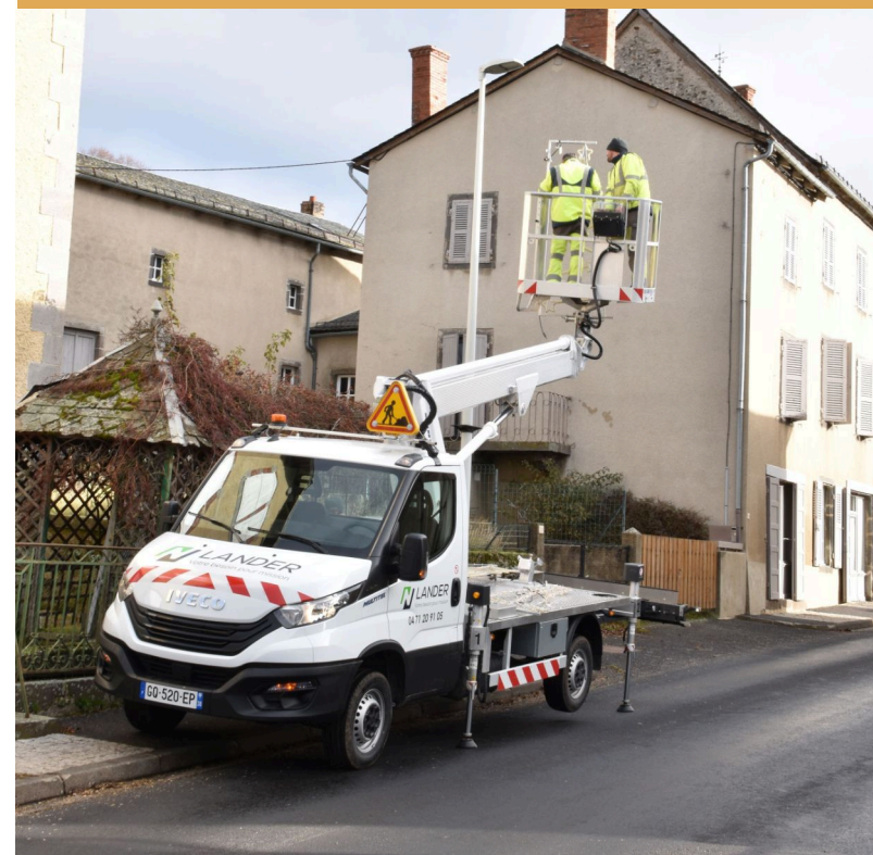
Installation des illuminations
